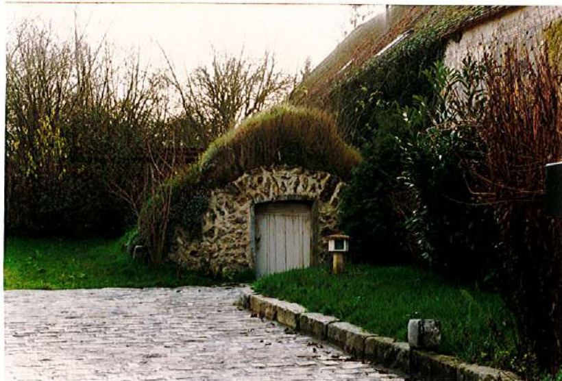
Cave semi-enterrée - Moutiers
